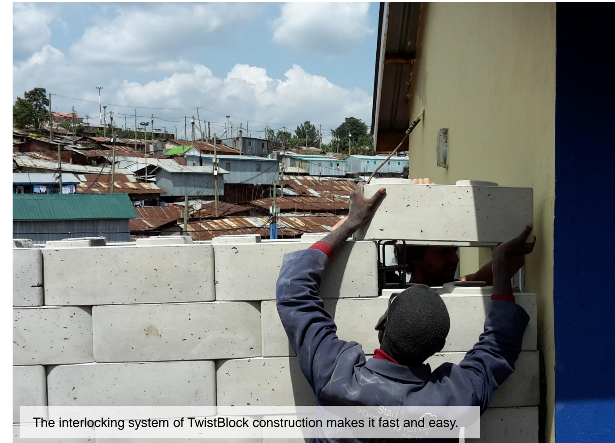
TwistBlocks are hollow and light weight and measure 175 x 250 x 500mm
