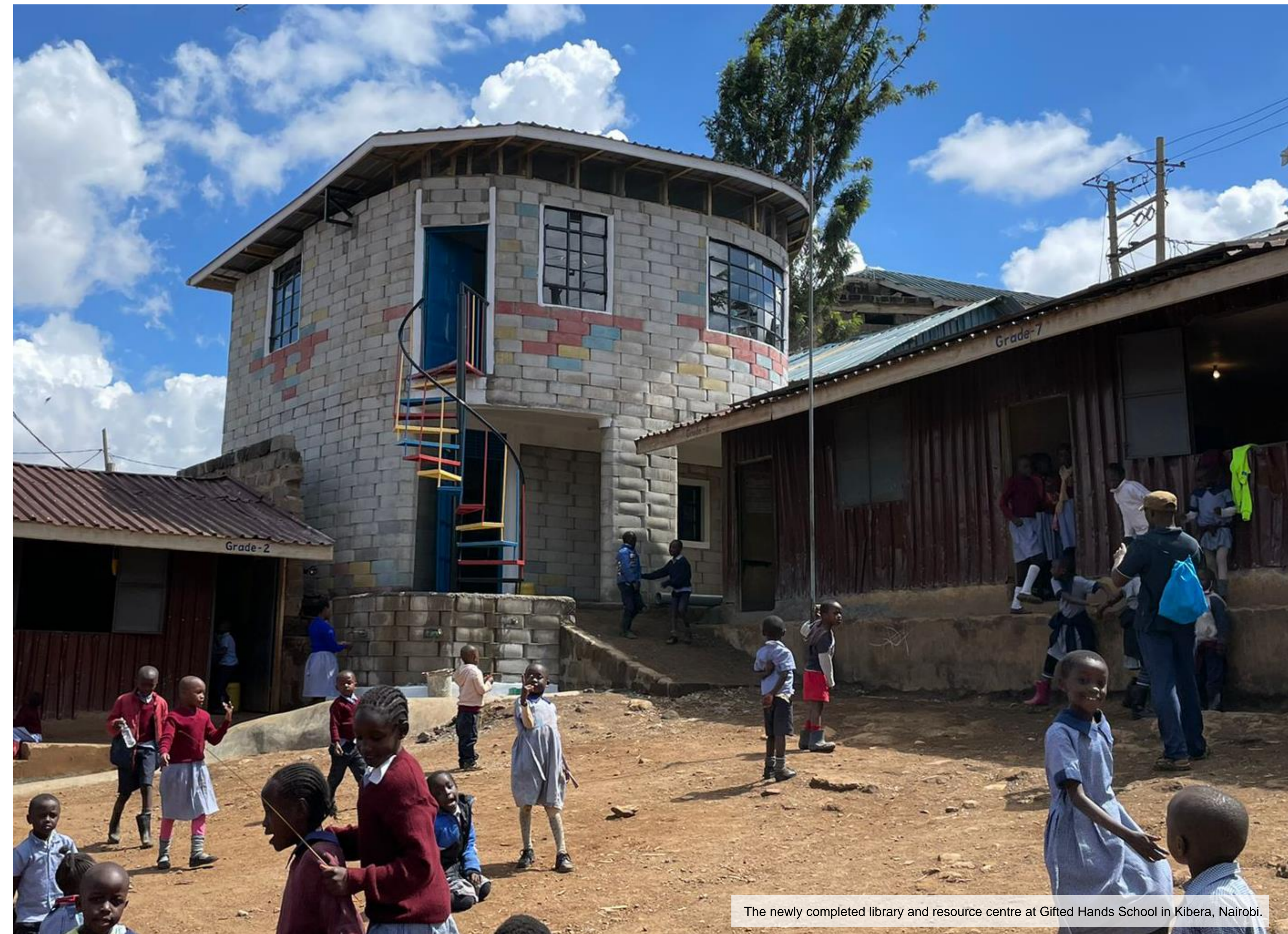
The interlocking system of TwistBlock construction makes it fast and easy.
